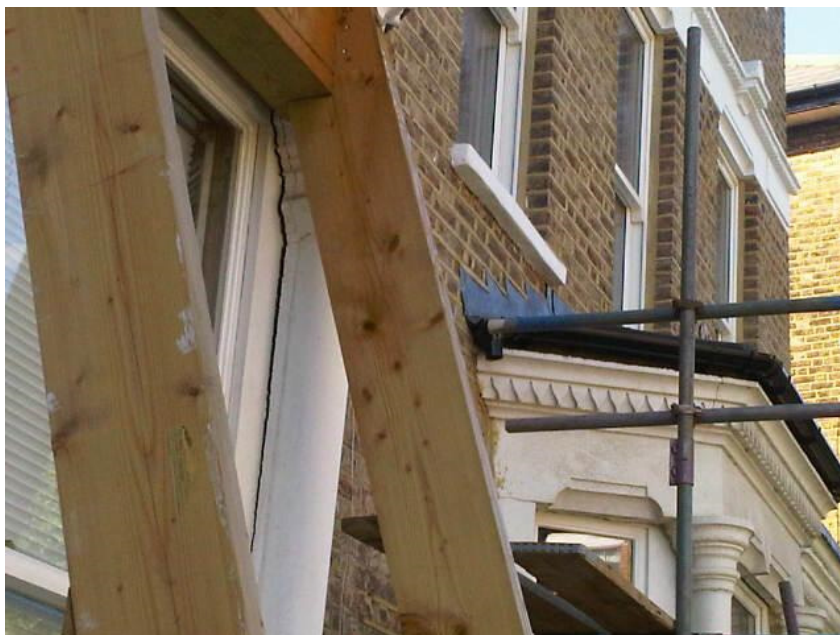
Cracked window frame and emergency structural support at 92 South Hill Park, caused by basement development next door
