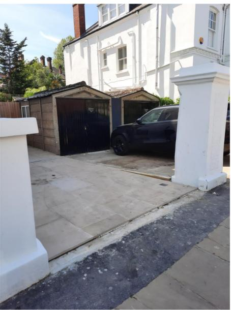
Original wall removed leaving isolated pillar not shown retained in drawings.
